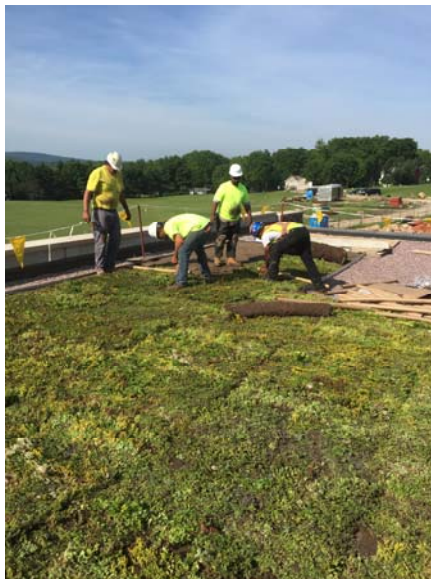
Sedum Mats being installed at the jobsite.
