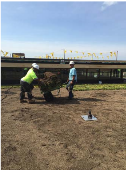
Rolled Sedum Mats being staged at the jobsite.
