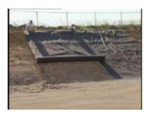
**Step 1**- Starting at the apex of the slope, deploy the geotextile downhill.
