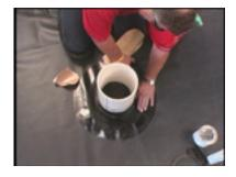
**Step 12**- Smooth the QuickSeam FormFlash down onto the Firestone EPDM Geomembrane panel.
