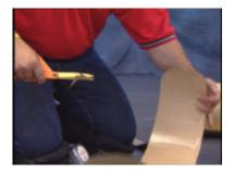
**Step 7**- Trim the corners of the FormFlash to remove any excess.
