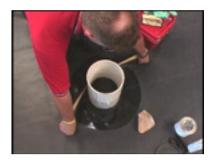
**Step 10**- Adhere the QuickSeam FormFlash to the flashing around the pipe.
