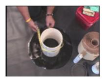
**Step 5**- Measure the diameter of the pipe and add 3" (7.62 cm) to determine the desired length of FormFlash.
