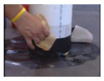
**Step 11**- Remove the plastic release film.
