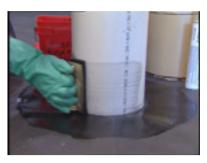
**Step 3**- Apply QuickPrime Plus Primer on to the pipe.
