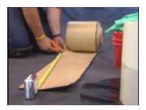
**Step 6**- Cut a length of 9.00" (22.86 cm) QuickSeam FormFlash that is long enough to extend around the pipe, overlap the base, and itself by several inches.
