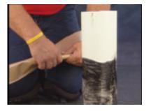
**Step 8**- Fold the FormFlash together along the length of the center perforation.
