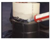
**Step 16**- Apply a continuous bead of Lap Sealant HS or All Purpose Sealant over the top edge of the boot and the edges of the base of the boot.
