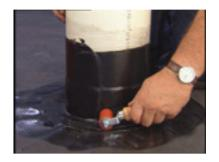
**Step 13**- Roll the pipe boot base flange on the Firestone EPDM Geomembrane panel and the flashing adhered to the pipe.
