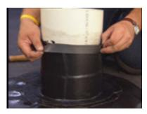
**Step 14**- Prior to tightening the stainless steel clamp around the FormFlash, you will need to protect the FormFlash. To do this, add a piece of scrap membrane to the area to be secured by the stainless steel clamp. This will reduce the damage to the FormFlash during the tightening process.
