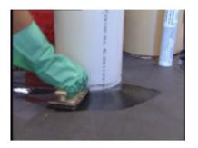
**Step 2**- Using a scrubber pad and holder; apply QuickPrime™ Plus Primer to an area around the pipe's base. Extend the primer coverage beyond the width of the pipe boot flange.
