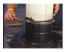
**Step 15**- Place the clamp over the FormFlash and tighten it. Cut away excess metal.
