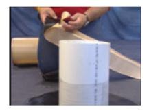
**Step 9**- Remove the release paper on one side of the folded-over flashing.
