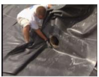
**<u>Sub Step 2</u>**- Cut a target patch with a properly sized hole and place it over the pipe.
