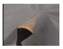
**<u>Sub Step 1</u>**- Cut the panel to expose the pipe.
