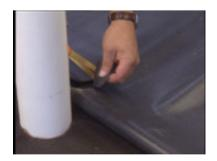
**Step 1**- Cut a hole in the Firestone EPDM Geomembrane panel that is approximately 75% of the outside diameter of the pipe protruding from the substrate.
