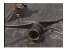
**Sub Step 3**- Ensure the liner is dry and free of mud and other contaminants.
