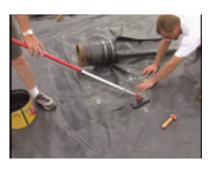
**Sub Step 4**- Seam the target patch to the Firestone EPDM Geomembrane panel with primer and either 6.00" (15.24 cm) QuickSeam™ Cover Strip or 3.00" (7.62 cm) QuickSeam Splice Tape
