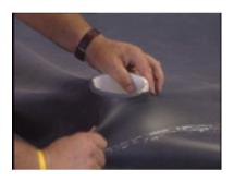
**Step 2**- Then, slide the membrane into place over the base of the pipe.
