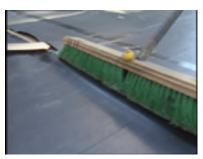
**Step 10**- Use a broom to brush over the splice to solidify the adhesion. Check for fish mouth folds and smooth out as necessary.
