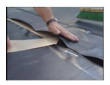
**Step 9**- Expose 0.25" to 0.125" (0.64 to 0.32 cm) of the tape outside the overlap. Remove the release paper and allow the top Firestone EPDM Geomembrane panel to fall across the tape while pulling the release paper away at a 45° angle.
