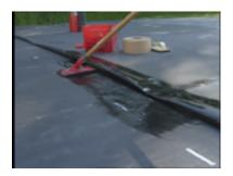
**Step 5**- Using a scrubber pad and holder; apply the QuickPrime Plus Primer to the bottom surface of the top panel and the top surface edge of the bottom panel.
