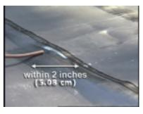
**Step 12**- Using a compressed air source, test all bonded seams using a minimum 50 p.s.i. (344.74 kPa) air supply directed through a 0.1875" (0.48 cm) nozzle held within 2.00" (5.08 cm) of the seam edge.
