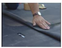
**Step 4**- Tack-back the overlap of the top Firestone EPDM Geomembrane panel using QuickPrime<sup>TM</sup> Plus Primer as an adhesive.
