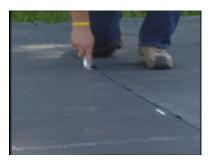
**Step 3**- Mark the overlap with a white marker to ensure the membrane returns to this placement after priming.
