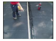
**Step 8**- Check the QuickSeam Splice Tape alignment to avoid "fish mouths" or folds in the tape.
