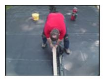
**Step 7**- Adhere the 3.00" (7.62 cm) QuickSeam Splice Tape to the primed surface of the bottom panel.
