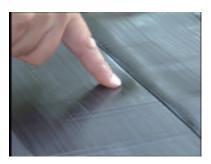
**Step 6**- Test the primer flash-off by touching the primed area with your finger and pushing forward at an angle. The primer should not string as your finger is moved up and away.
