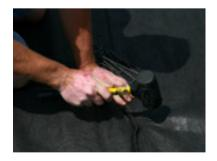
**Step 1**- Use sod staples to hold the geotextile in place.
