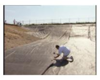
**Step 2**- Remove all bent or excess staples that pose a hazard of puncturing the Firestone EPDM Geomembrane.
