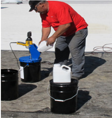
Mix Part B with Part A for three minutes. Add Part B slowly to part A
