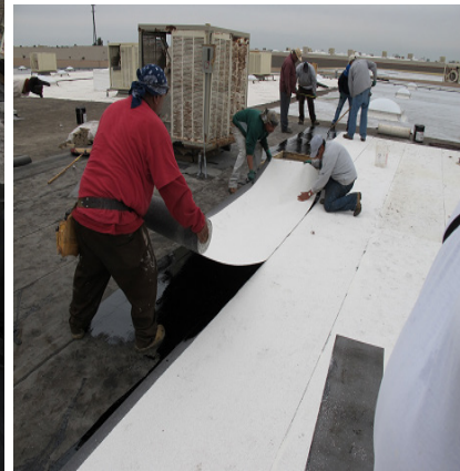
Lay Cap Sheet in adhesive
