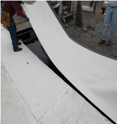
Lay Cap Sheet in adhesive
