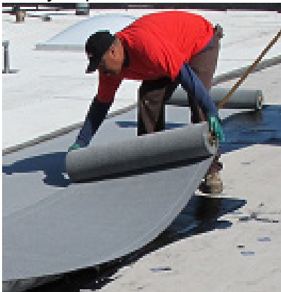
Lay Base Sheet in adhesive
